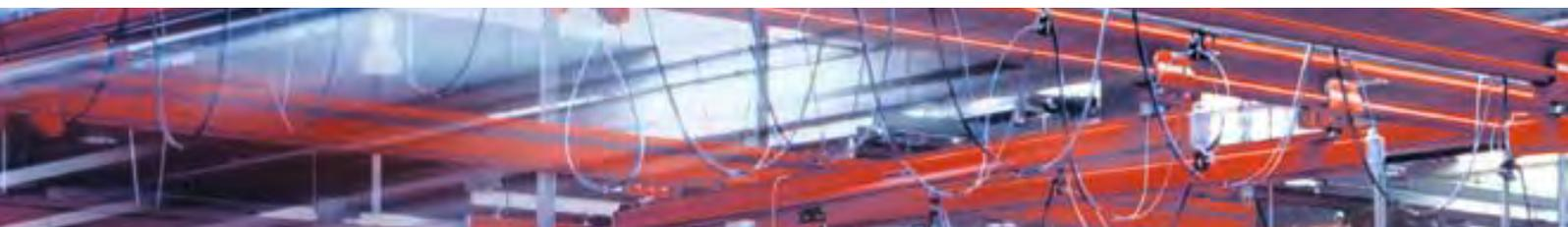
Different profile section sizes can be used for single and double-girder suspension crane runways and girders. All components are protected against corrosion – they are either finished with a coat of paint, galvanised or coated with KTL.
